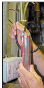
Furnace draft (left)
