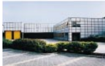
European Headquarters and Manufacturing Facility, High Wycombe, Bucks, England
