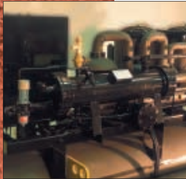
shell & tube condenser
